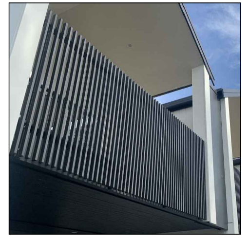
BALUSTRADE 50 X 20mm RHS ALUMINIUM BATTEN BALUSTRADE WITH MAX 70mm SPACINGS POWDERCOAT FINISH
