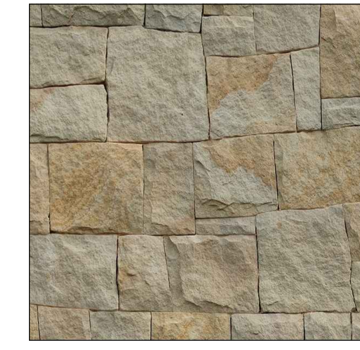
SITE WALLS MIN 50mm DRY JOINT ROUGH SANDSTONE CLADDING FIXED TO CONCRETE SUBSTRATE
